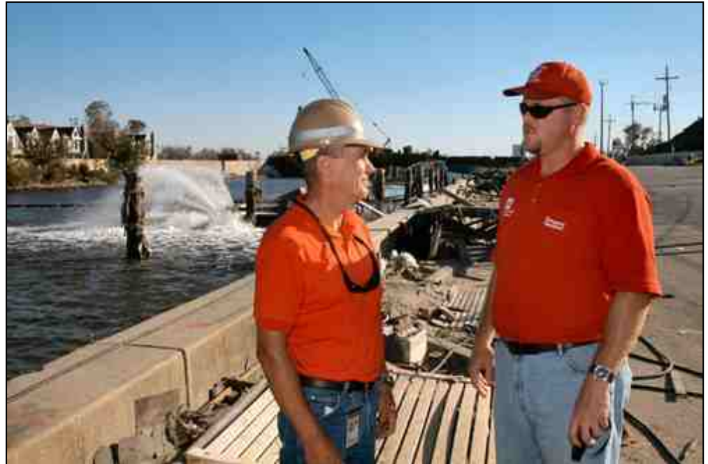
New Orleans District employee Casey Rowe (r), environmental resources specialist, gives coworker Edward Wrubluski, quality assurance representative, an overview of the aerators on the 17 th Street Canal. The aerators put oxygen back into the water to avoid fish kills and to keep organic matter decomposed. Photo by Alan Dooley, St. Louis District
